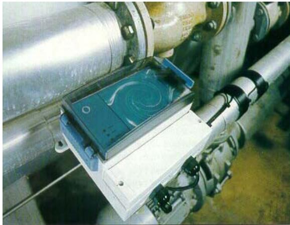
**Fig 4: A typical *Scalewatcher* installation. Note the tightly wound coils in the centre right of the photo.**
