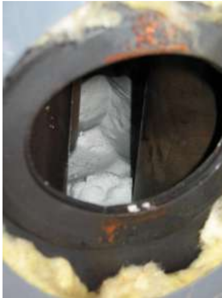
Installed 02/21/07 – room #27 still in service
